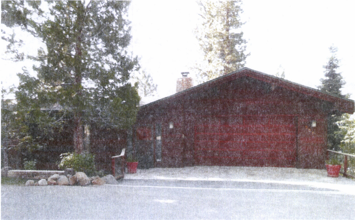
557 Dale Drive (Subject property). The front door on the left extending two feet beyond the garage face.
