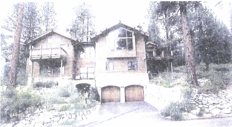
Retaining wall on right requires variance for entry
