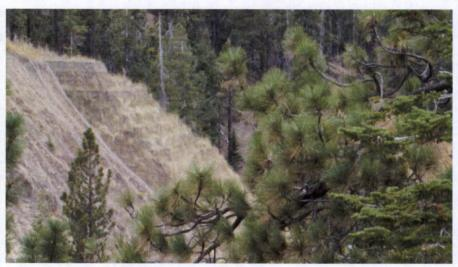
Terraced and planted rock cuts such as those used on US 50 in Lake Tahoe are preferred over the use of rock fall protection fencing.
