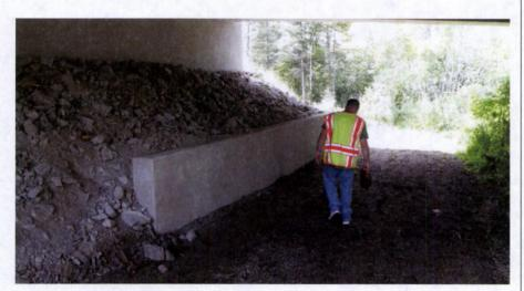
Facilitate movement through wildlife passages by utilizing natural surfacing. The crossing may be coordinated with creek crossings when appropriate. The natural streambank should be maintained through the structure.
