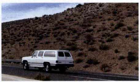
Naturalized rock cuts and grading that blend with the surrounding topography are preferred. Mass grading of slopes is visually unappealing and leads to vegetation management issues.
