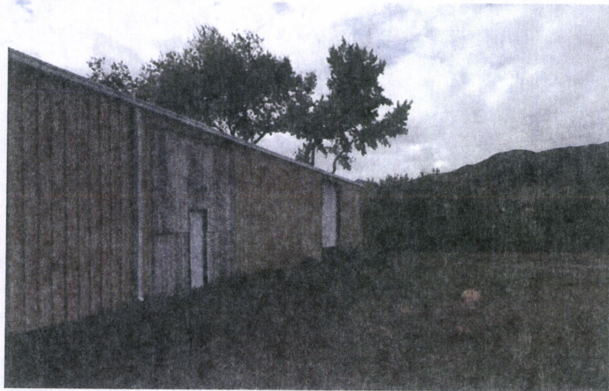
Existing industrial building
