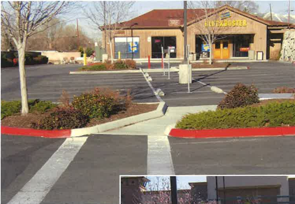
Photo A-1: Pedestrian Walkways within Parking Lots
