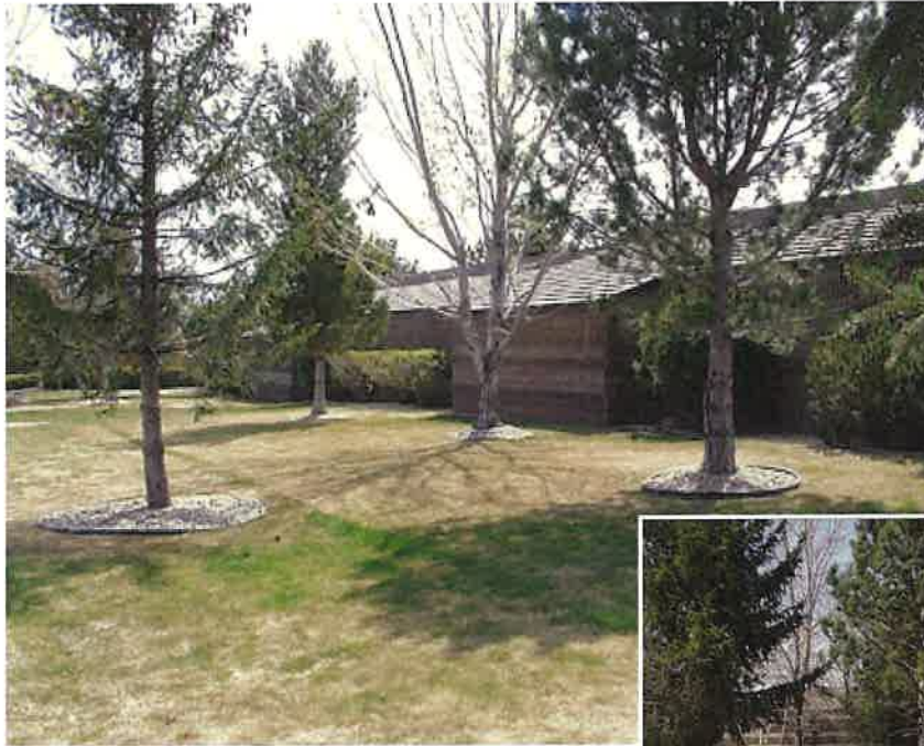
Photo A-3: Desirable Design Characteristics for Personal Storage Facilities
