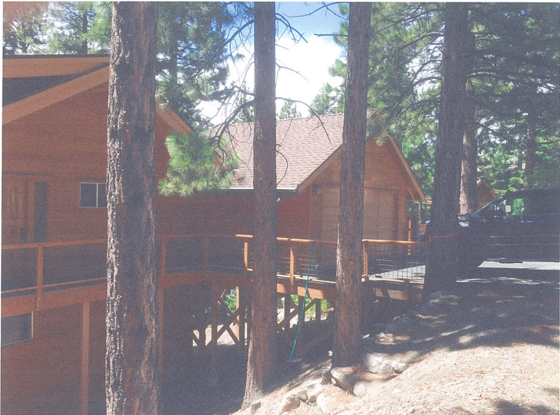
5. Photo facing the existing garage and front entrance to the residence.
