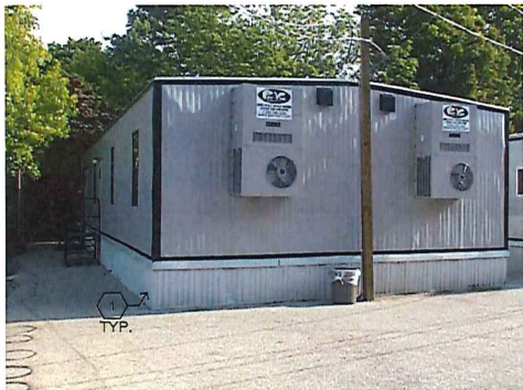
TYPICAL FINISHED MODULAR BUILDING W/ SKIRT
