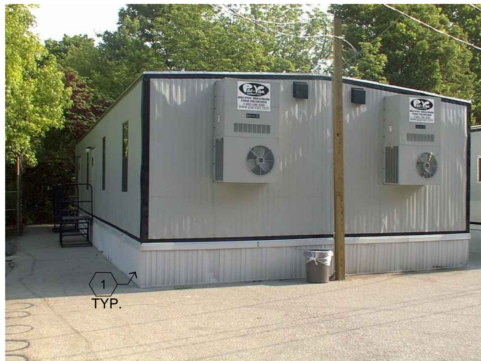
TYPICAL FINISHED MODULAR BUILDING W/ SKIRT
