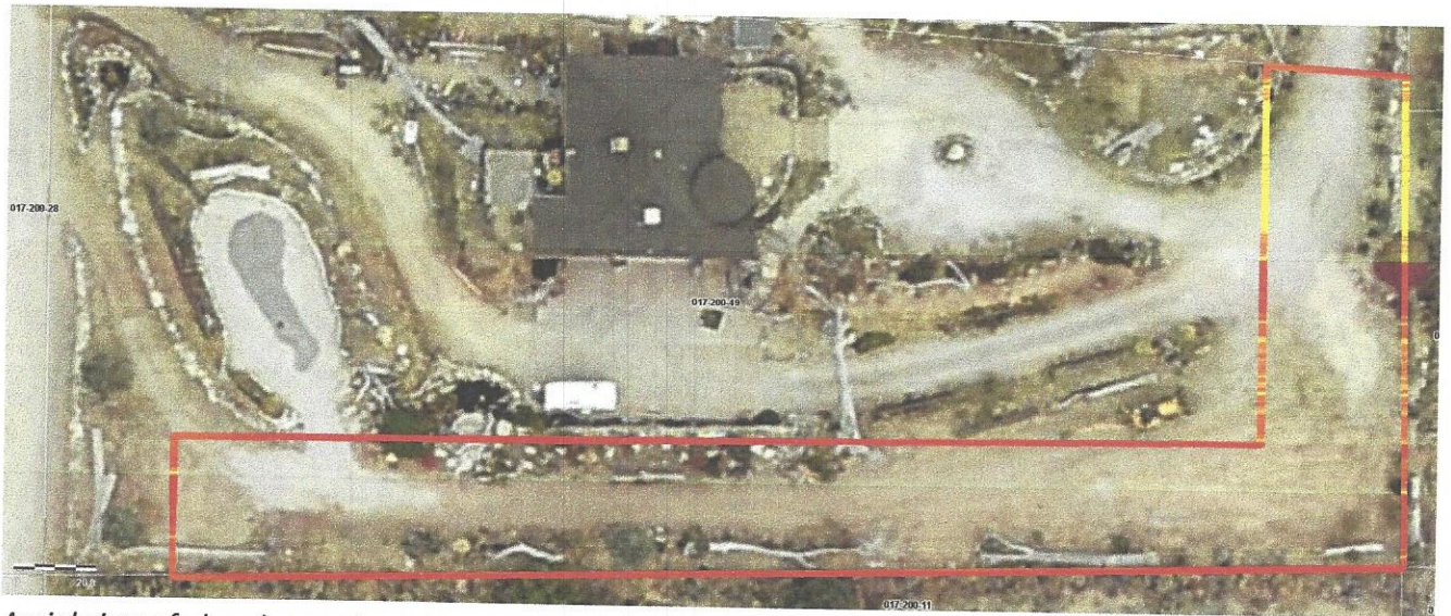
Aerial view of abandonment area
