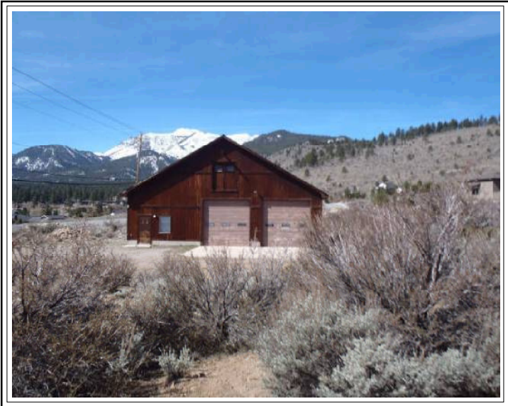
Front Shop, Office (East Side)
