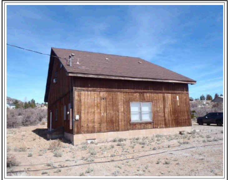
Back Side Shop, Office (South Side)
