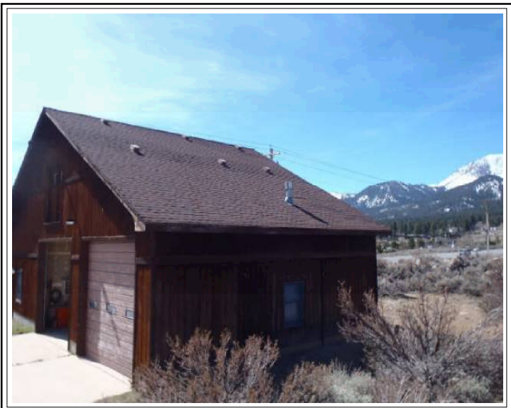
Front Side Shop, Office (North Side)
