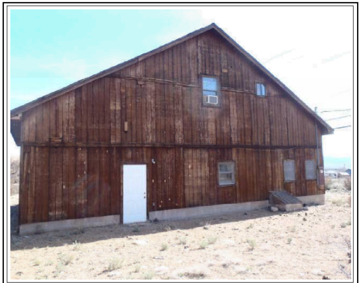
Rear Shop, Office (West Side)
