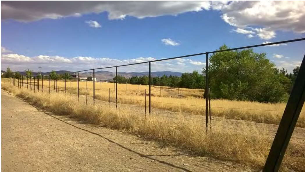
Phase III and IV of the fencing project at the north end of the Arboretum
