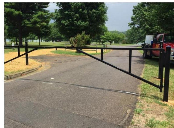
35 New Vehicular Gate (Manual)
