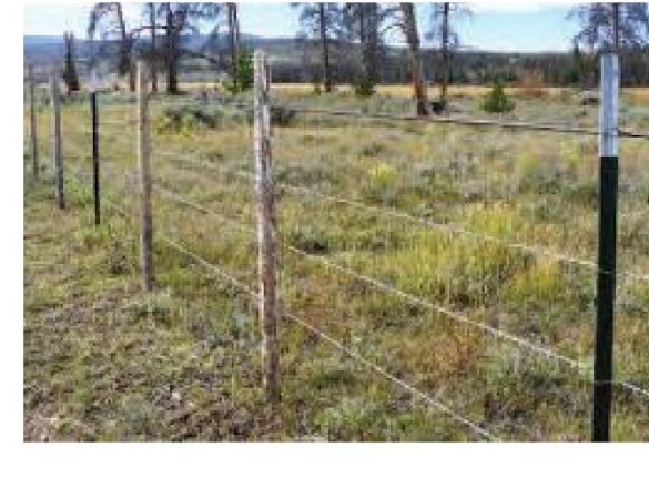
32 New/Upgraded Horse Exclusion Fencing
