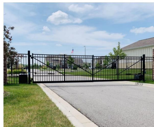
34 New Vehicular Gate (Automatic)
