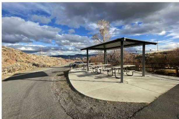
New Minor Shade Structure
