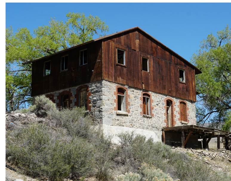
Avansino Ranch House
