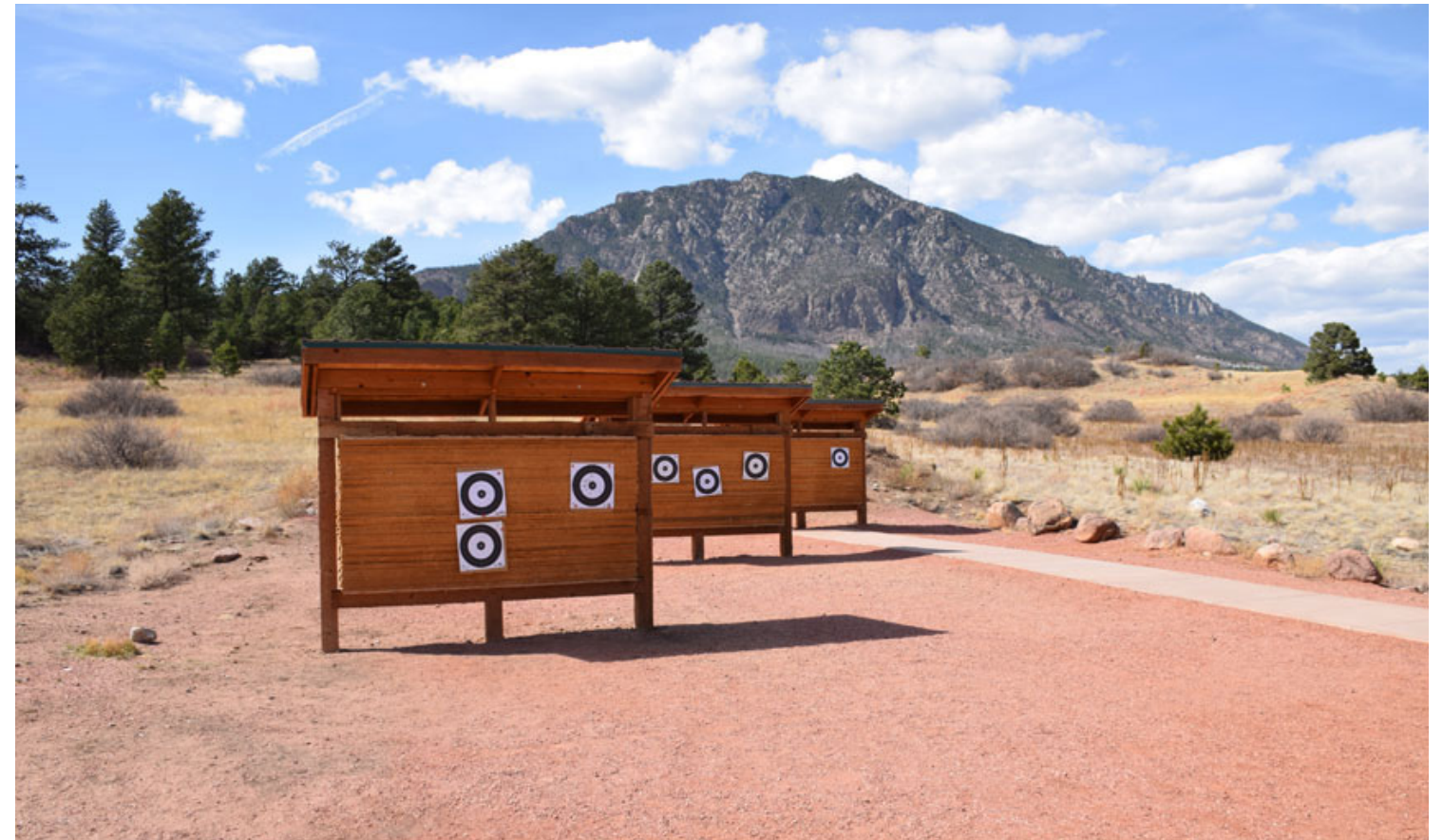
Regional Park, CO - Example of facilities.
